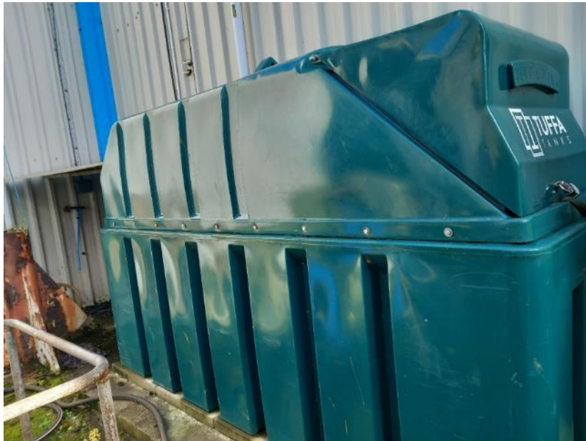
Photo 27. Diesel tank to the west of Building 45.
